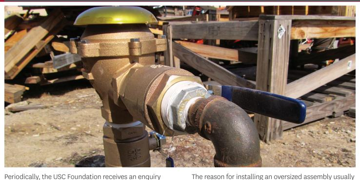
Periodically, the USC Foundation receives an enquiry regarding the oversizing of backflow prevention assemblies in a system. Some think that installing a larger assembly into a system with smaller piping reduces the pressure loss across the assembly, but even though the assembly will continue to provide backflow protection in this type of installation the reasoning for the installation may not provide the desired results.
